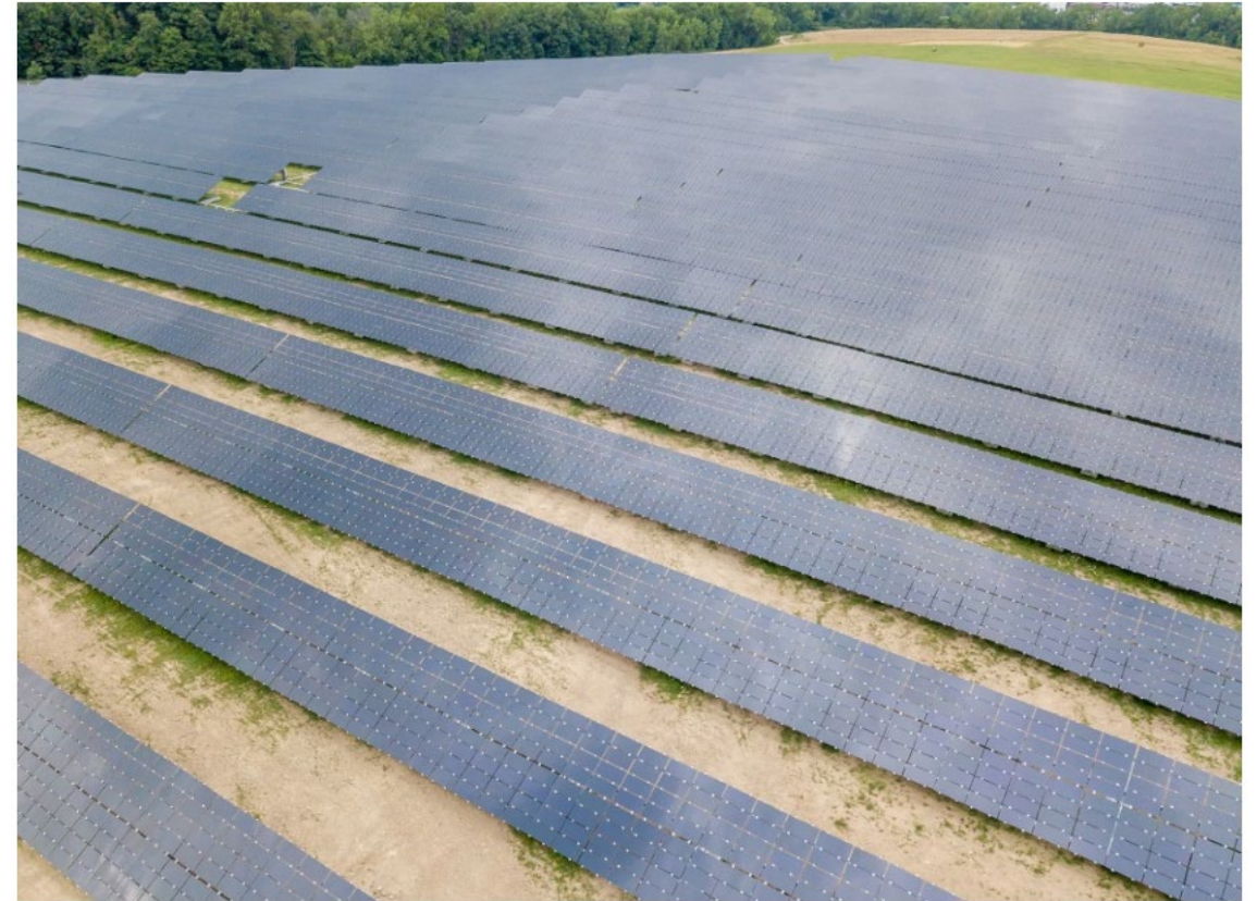
The old Brooklyn landfill is a new county solar farm [ Cuyahoga County Sustainability Office ]
